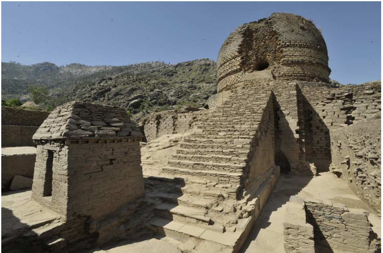
Figures 19 and 20. Amluk-dara: the Main Stūpa before and after excavation and restoration (Photo E. Loliva; copyright IAMP.)
